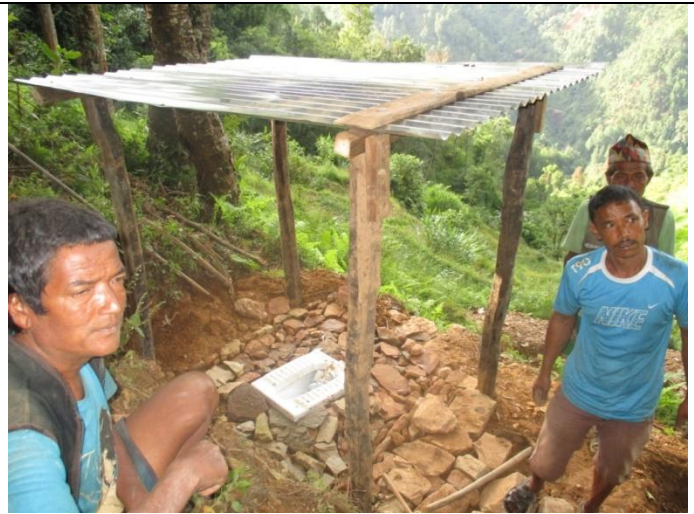
New constructed latrine
