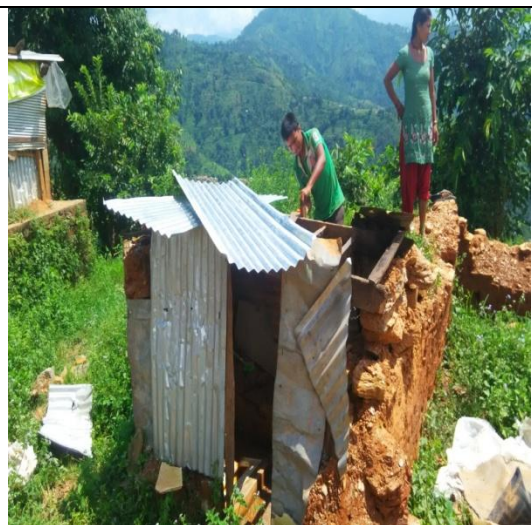
During Revival of Toilet
