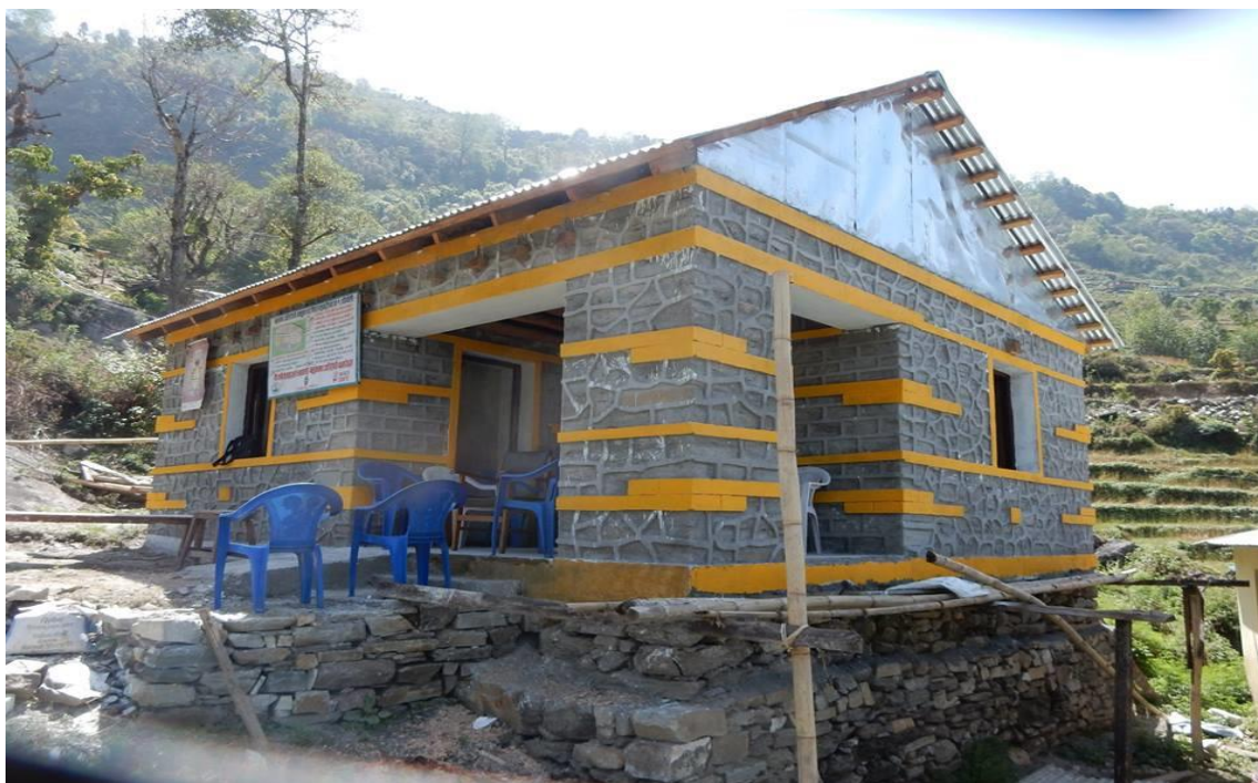
Fig: Demo House constructed in Ghorthali
