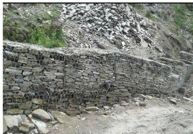
Landslide mitigation in Hagam
