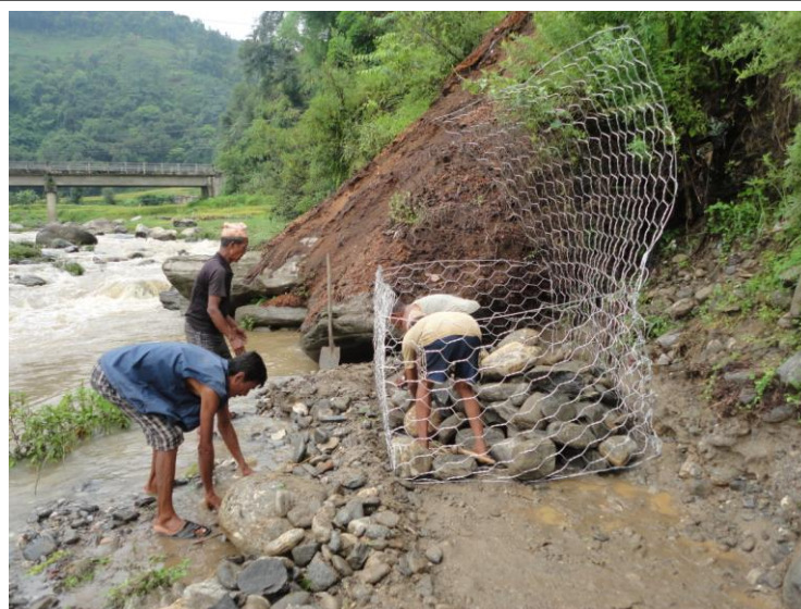
Photo: Farmers packing gabion box to protect agriland from river cutting
