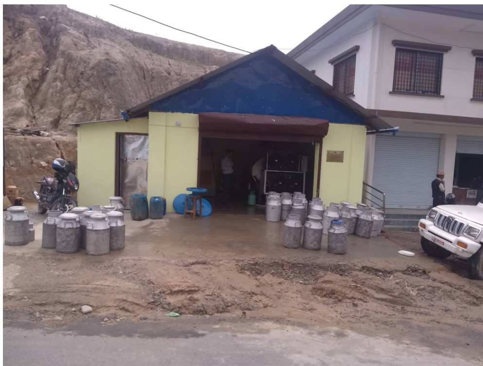
Figure 14 Bhotechaur Chilling Vat Building after opening.
