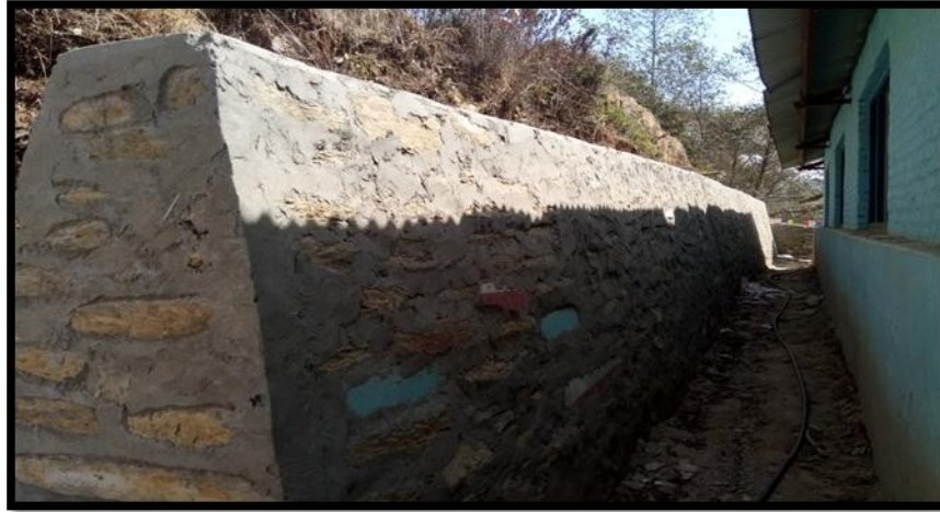
Stone Masonry Wall at Kakaling Harisiddhi Secondary School
