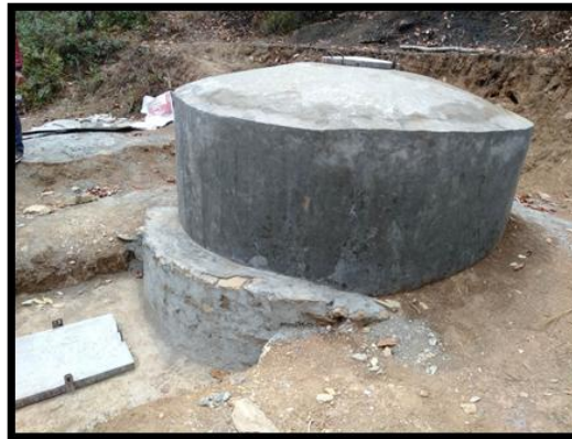
Ferrocement Tank at Sangme Water Scheme
