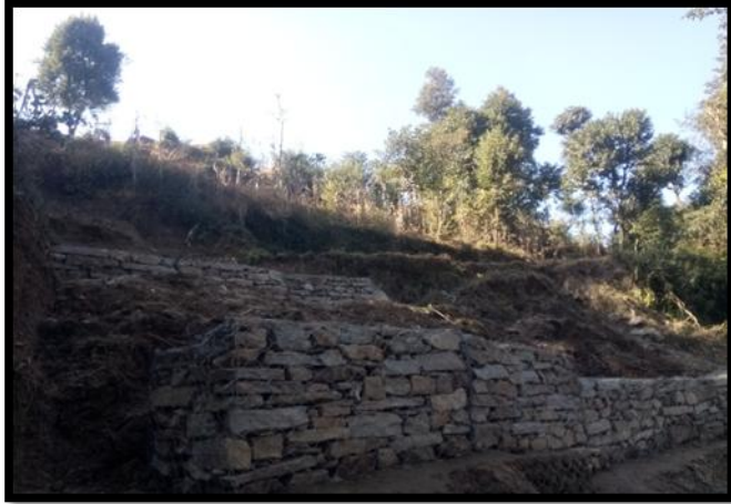
Gabion Wall at Khatrigaun Road
