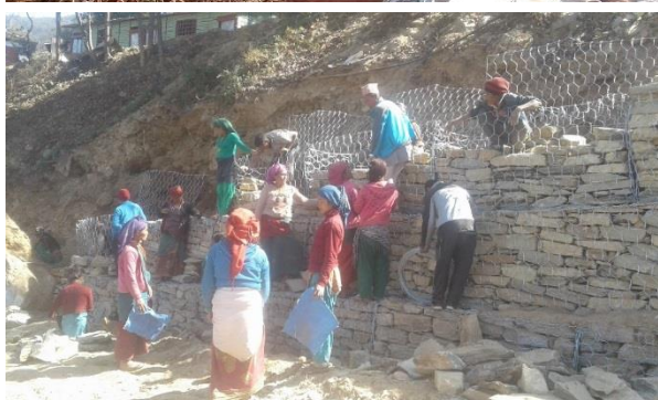
Figure 43: Beneficiaries Working on DR mitigation Site
