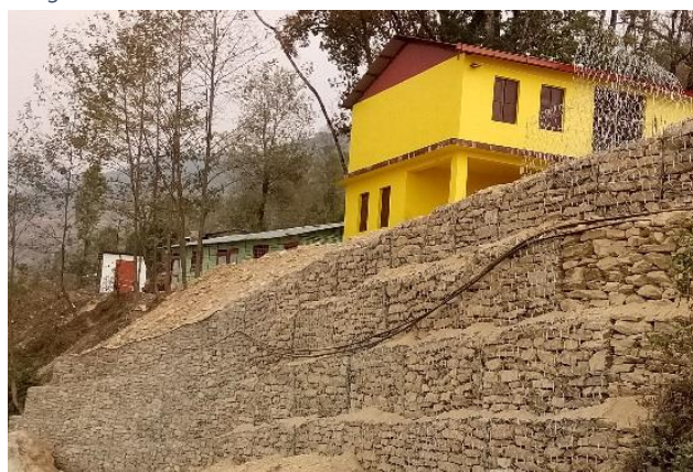
Figure 42: Disaster Risk Mitigation Work, Phulpingkot, Chyandanda School
